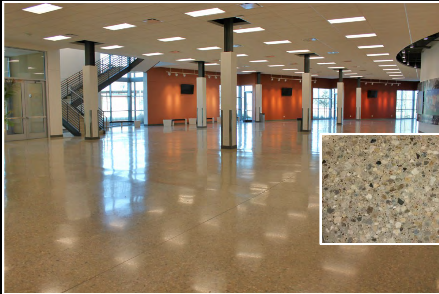
Project Location – Texas; Bomanite Custom Polishing System – Bomanite VitraFlor
