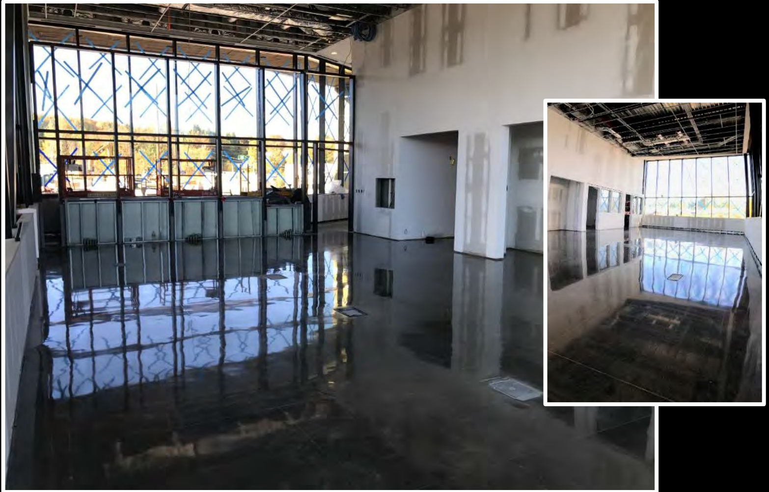
Project Location – Vermont; Bomanite Custom Polishing System – Bomanite VitrAFlor
