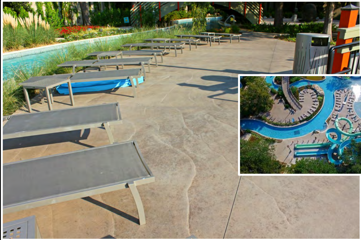
Project Location – Texas; Bomanite Imprint System – Pattern Erosion Series Shifting Sand Bomanite Exposed Aggregate System - Bomanite Sandscape Texture, Bomanite Sandscape Refined
