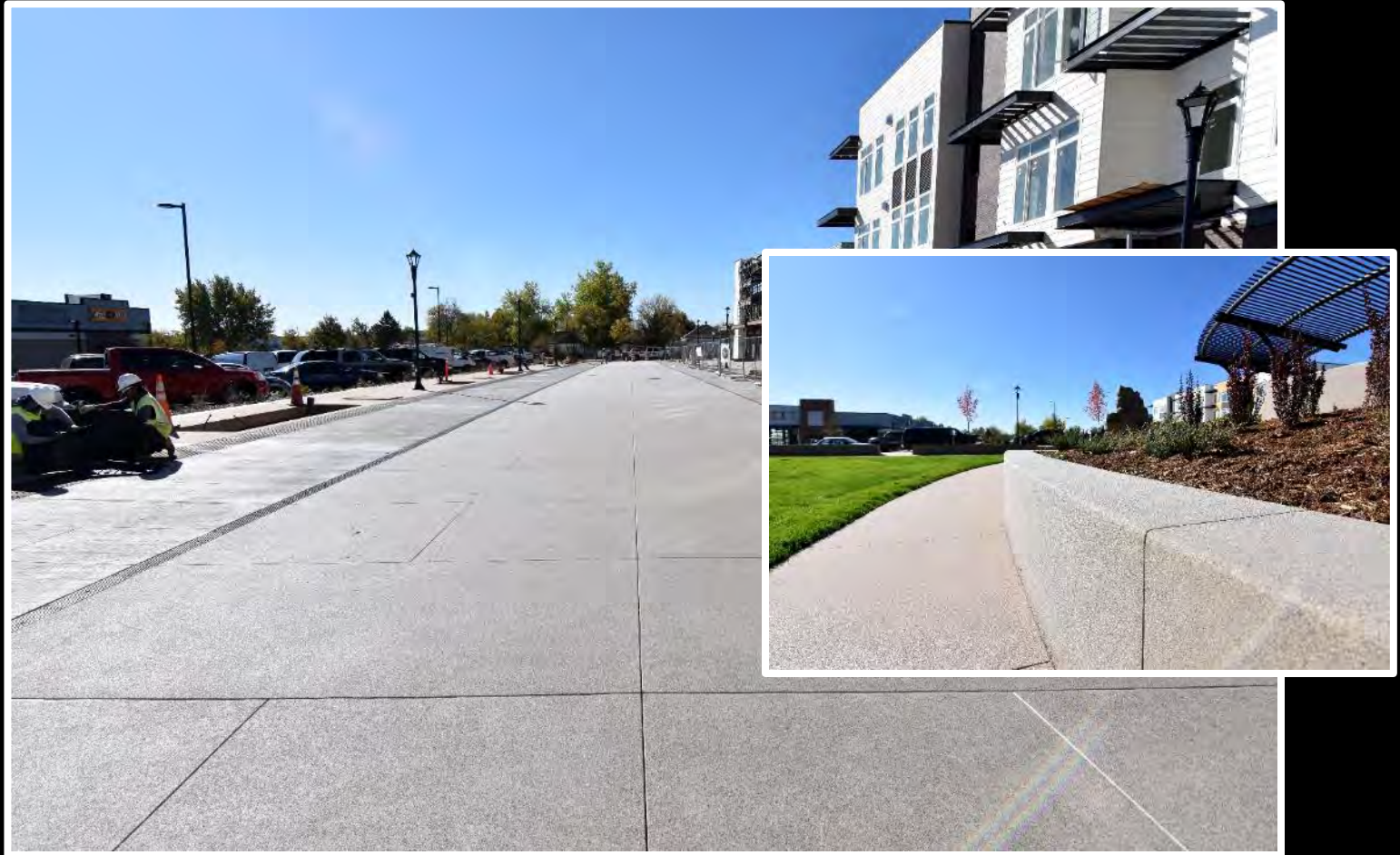
Project Location – Colorado; Bomanite Exposed Aggregate System – Sandscape Texture and Sandscape Refined
