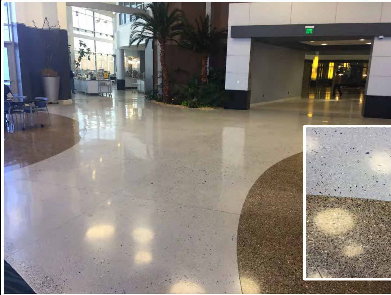
Project Location – Minnesota; Bomanite Custom Polishing System – Bomanite Modena Monolithic
